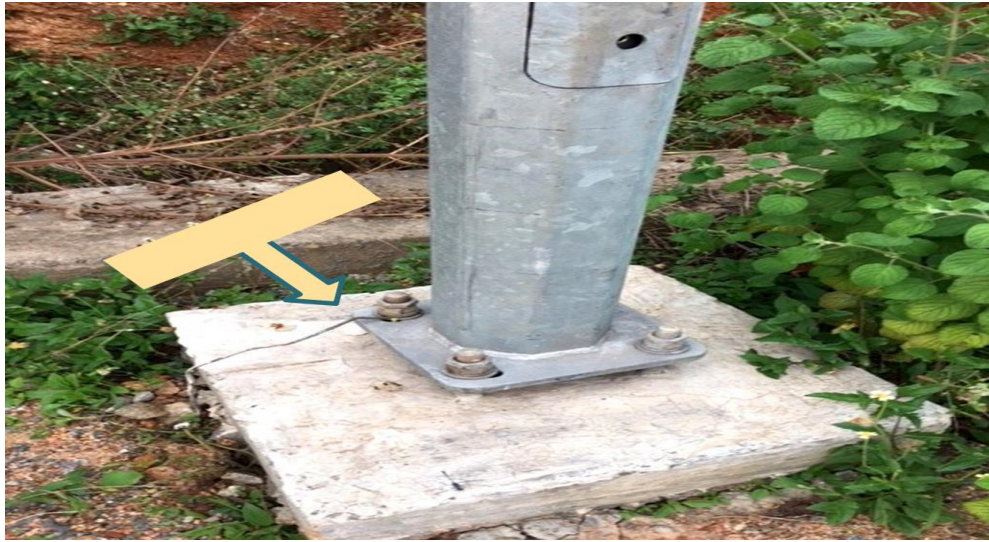
Fig.2.23. Strip Earthing
