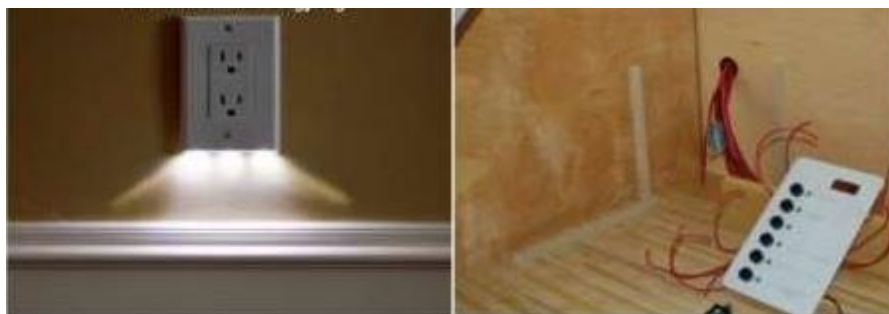
Fig.2.9. Concealed conduit wiring.
